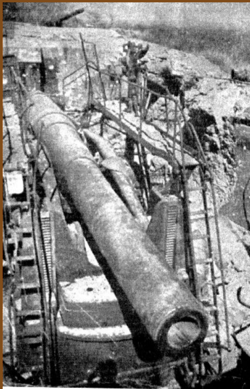
One of the large caliber guns on the fortress completely destroyed.
