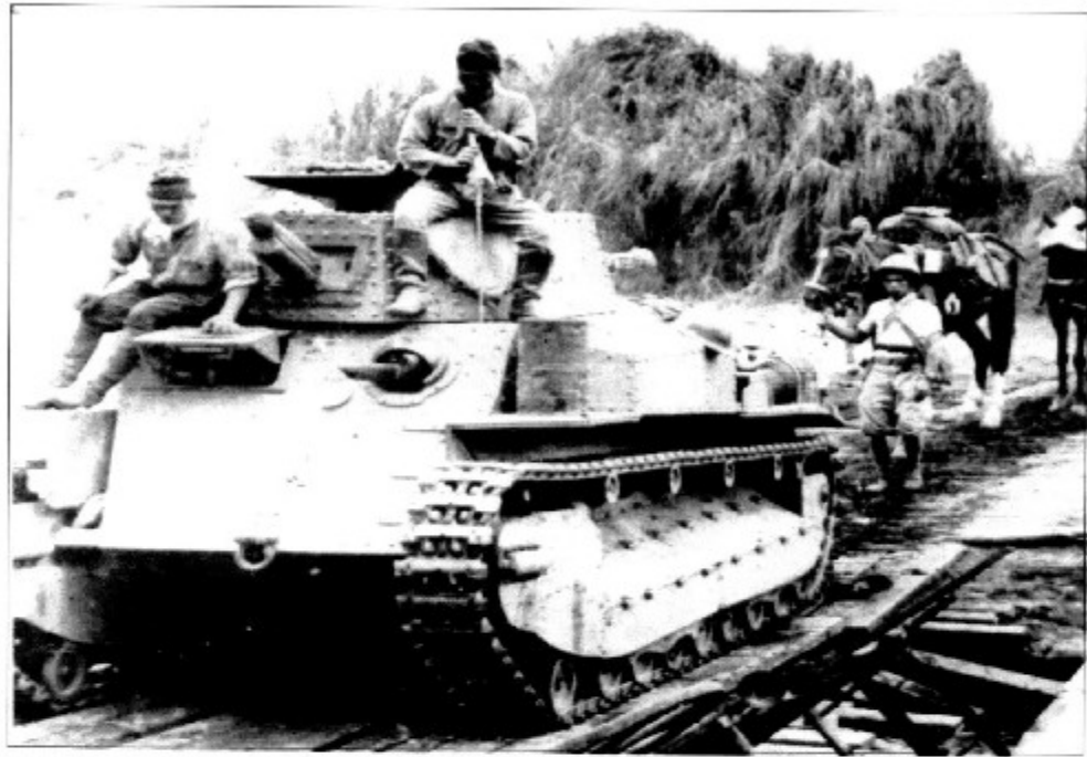
Japanese tank advancing towards Bataan..
