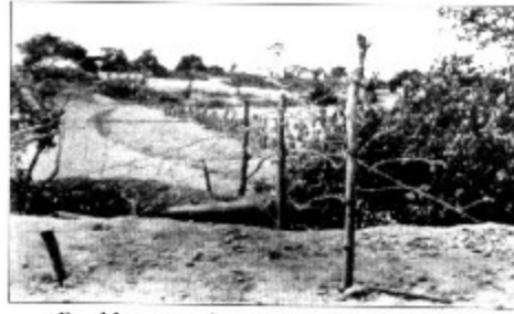
Double-apron fence entanglements set up.
