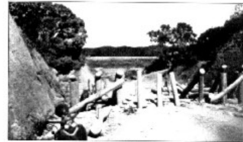
Tank obstacles and road blocks were constructed.
