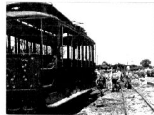
The heavily damaged transportation system.
